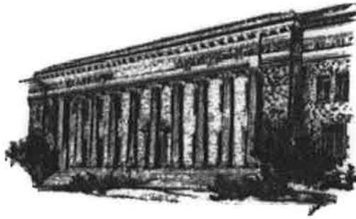
Tehama County Courthouse
